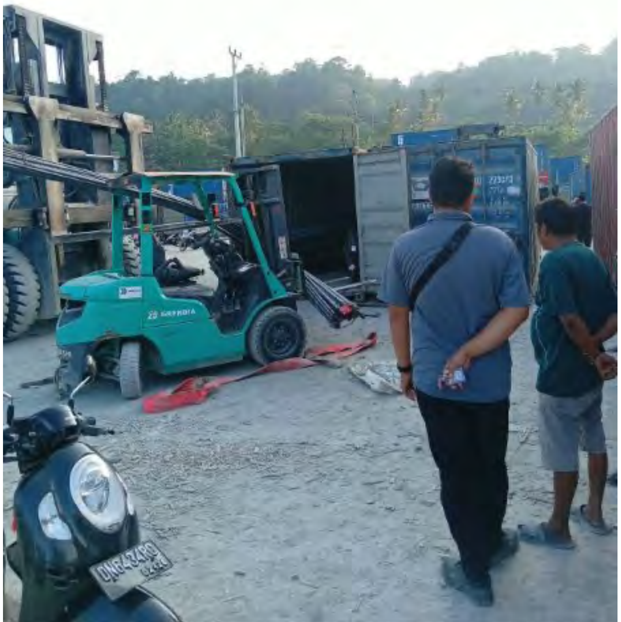
Kintom Police Chief, AKP Muh. Zulfikar, SH said that during the incident the victim was carrying out the work of unloading the threaded concrete iron from the container.
