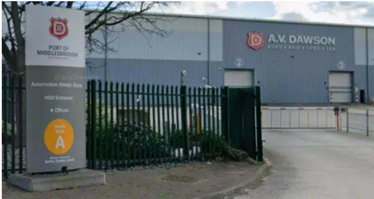
The worker dies at the AV Dawson site at Middlesbrough Port
