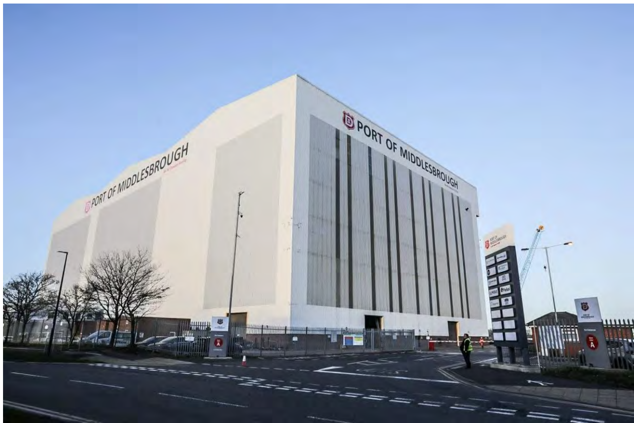
The Port of Middlesbrough, which AV Dawson owns and operates ( Image: STUART BOULTON )
