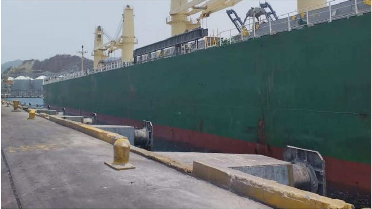
Pier 7 of the maritime terminal of Santa Marta.
