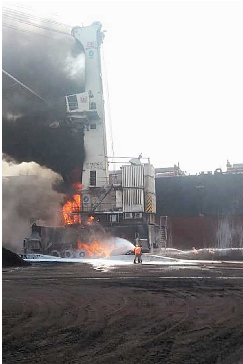
The crane on fire at Haldia port. Picture by Jahangir Badsa
