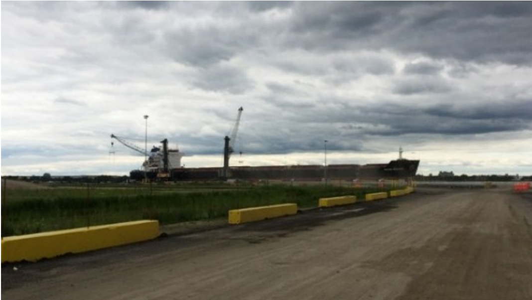
Bulker at the new Paulsboro Marine Terminal, 2017 (file image courtesy BP)
