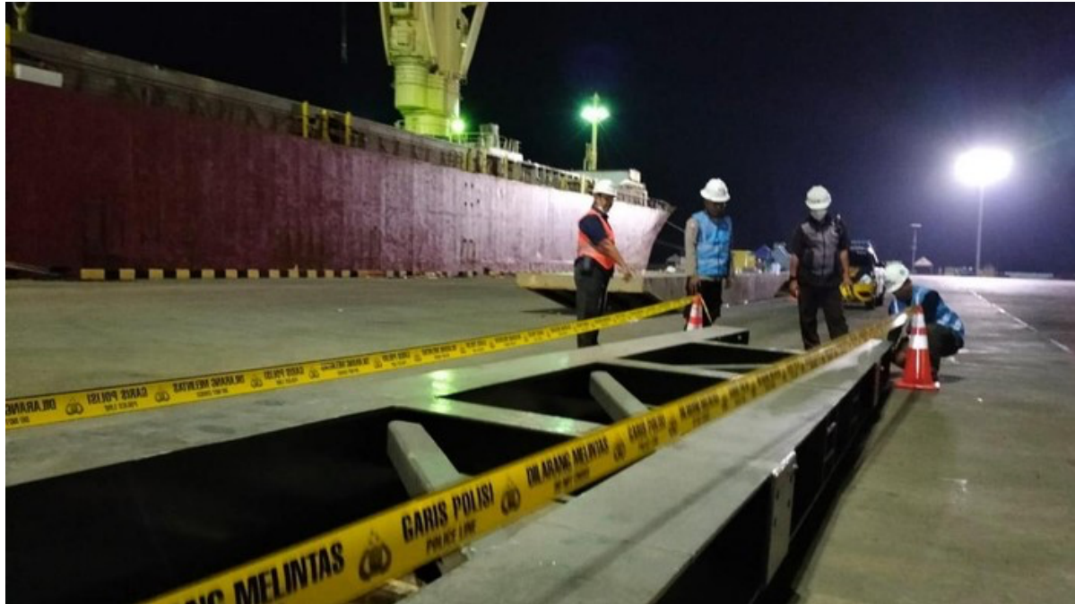
The location of the work accident at JIPE is installed with a police line. (Photo: Special/Reskrim Gresik Police for detikJatim)
