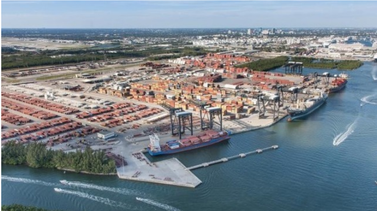
Cargo terminals at Port Everglades (file image)
